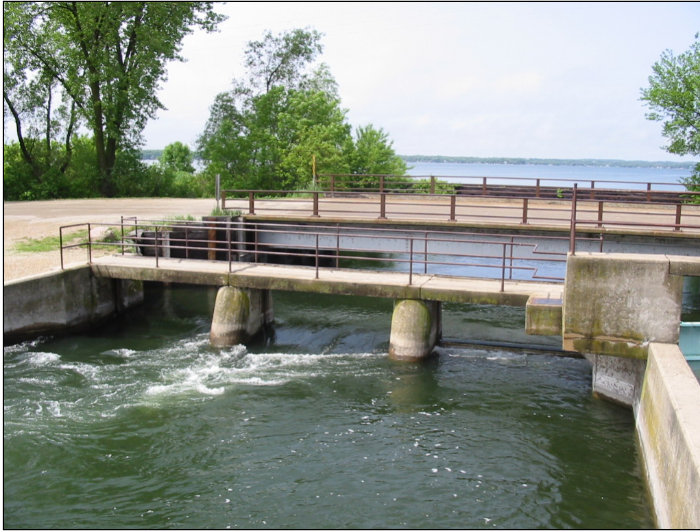
Figure 8. Dam at Lafollette County Park, Outlet from Lake Kegonsa
