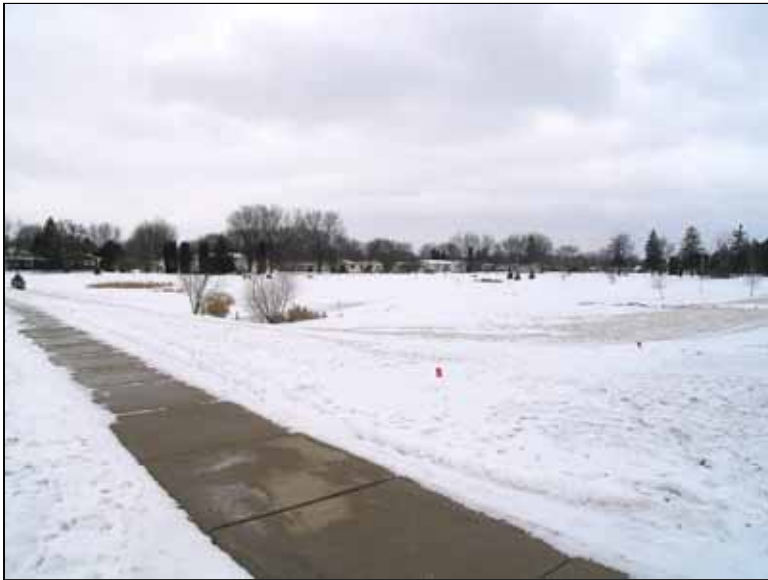
View of regional stormwater Pond (Silent St. Pond) west of Enterprise Drive.
